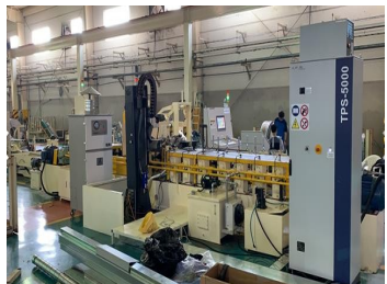
LASER Welding Pipe
